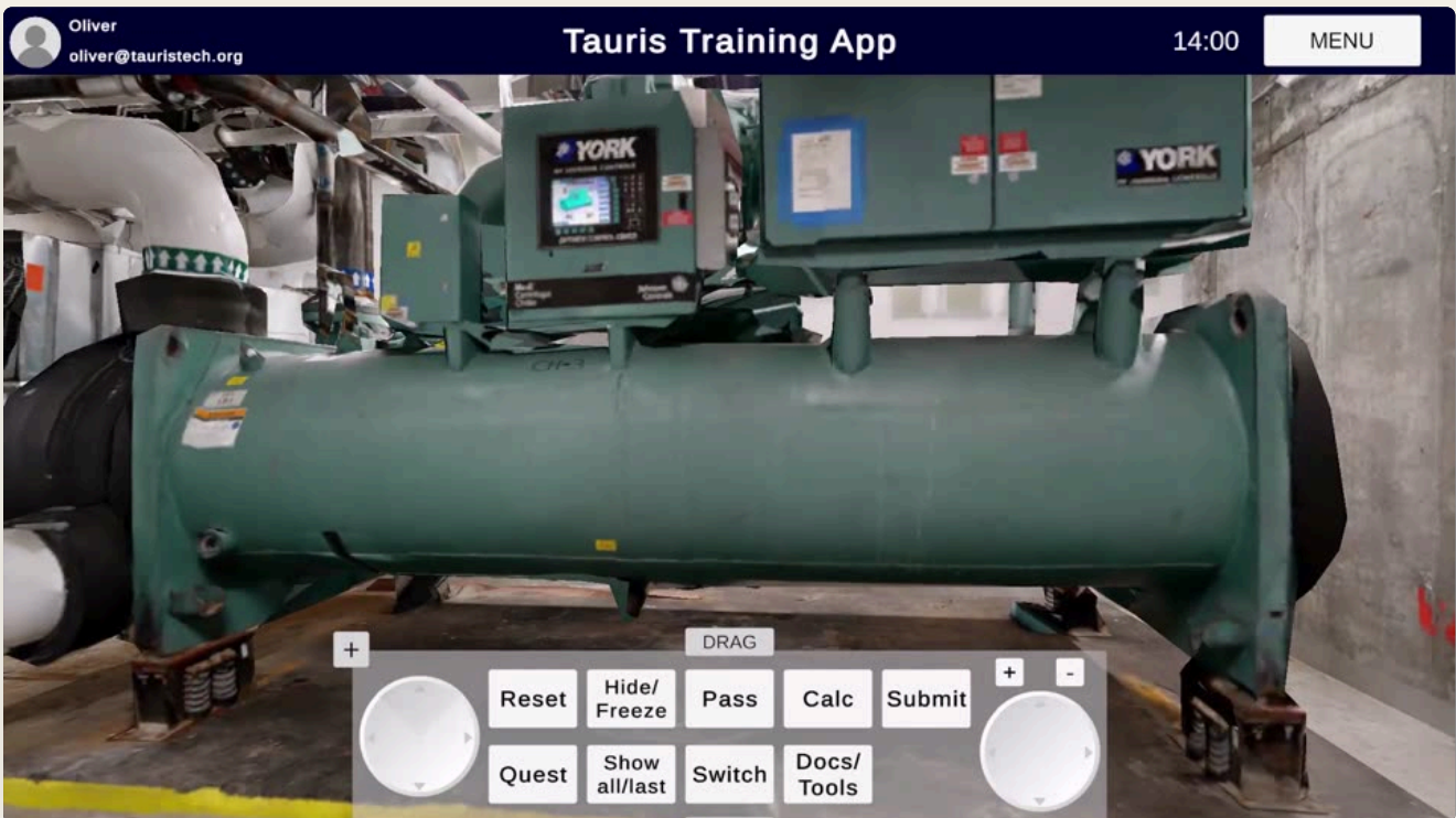
FIG. 03.1 Centrifugal chiller – simulator wide view
